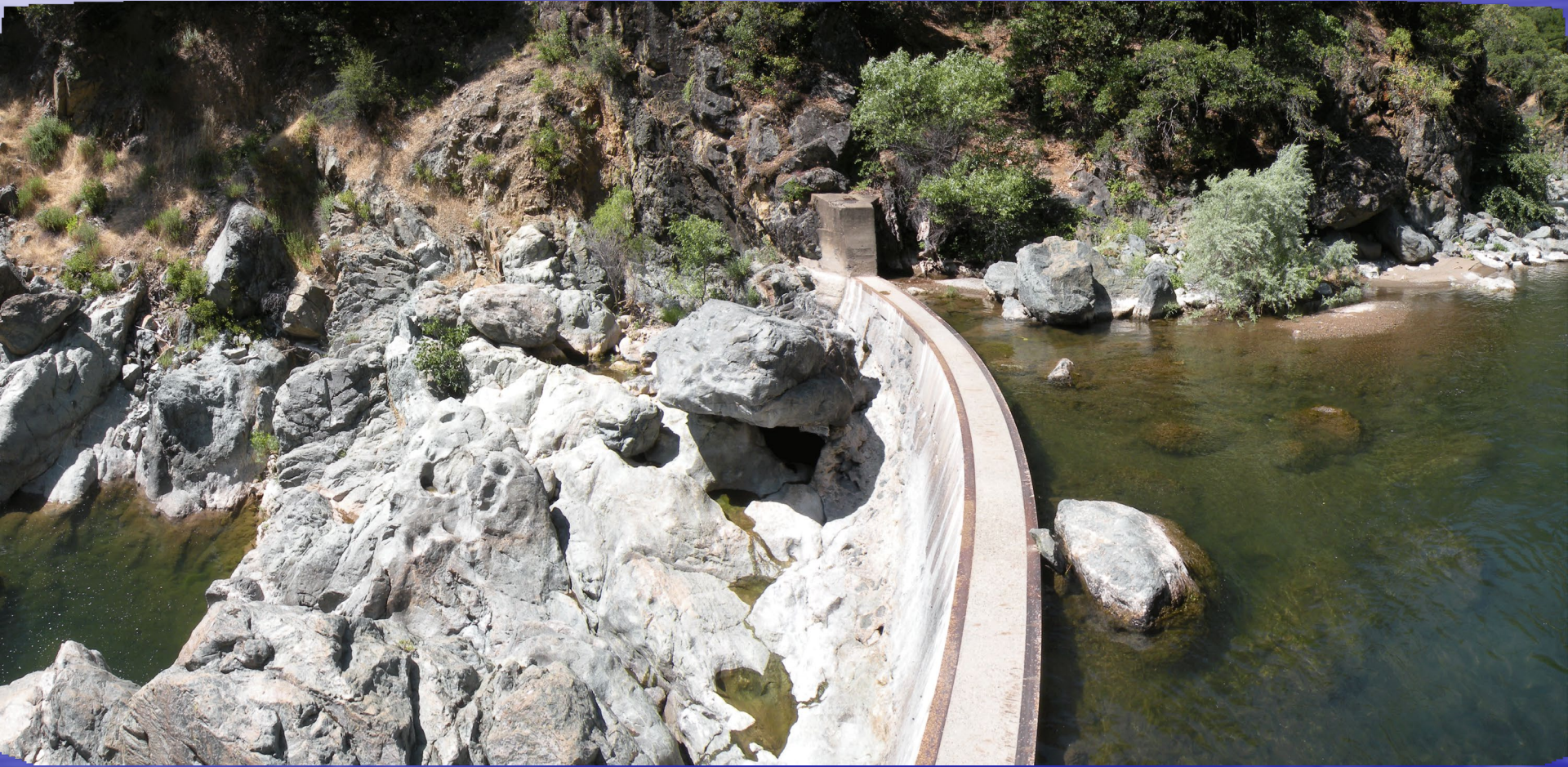
Centerville Head Dam 1150 feet elevation
